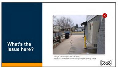
Avoid Installing outdoor units on walkways and patios Defrost cycle melt water can re-freeze on ground surfaces and create a dangerous slip hazard.
