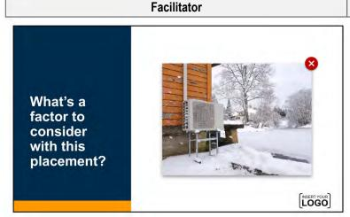
Don't install outdoor units facing into the wind If the outdoor unit is facing into dominant wind direction, this could cause counterrotation of the outdoor fan and lead to failure of the fan motor, fan circuit board or both.
